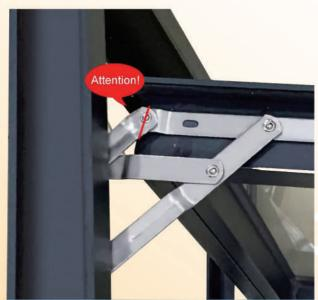
When the rivet at the top of the hinge exposes about half of the window sash, mark the corresponding hole spacing.
