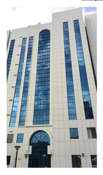
Smart Architectural Systems façade systems are designed with a 50 mm wide mullion and transom that is easily fabricated and assembled.
